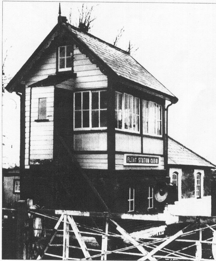
A typical MGWR signal cabin at Float on the Cavan line, photographed shortly before the branch closed. Although this cabin has external steps many had the steps placed internally for added security. Also typical are the Midland pattern crossing gates. Author's collection.
